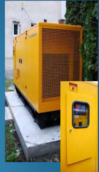
Power generator 275kW
