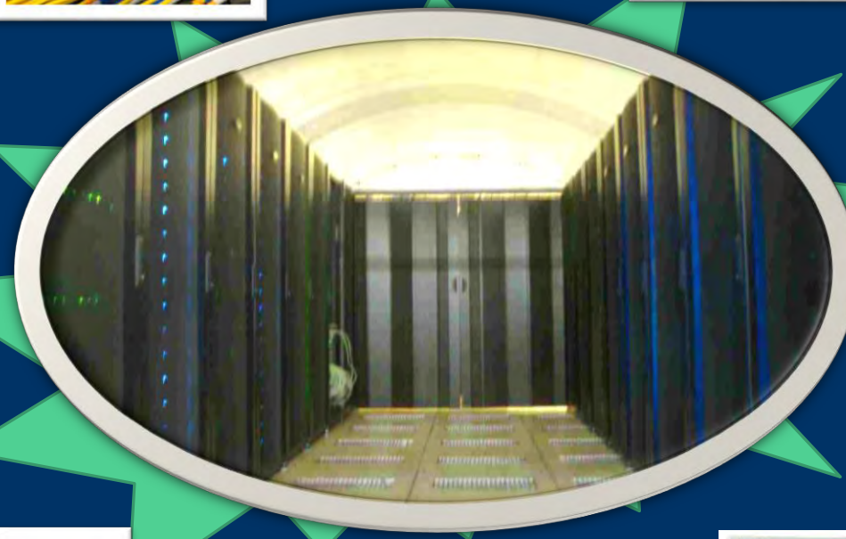
High Density Heat Containment System
